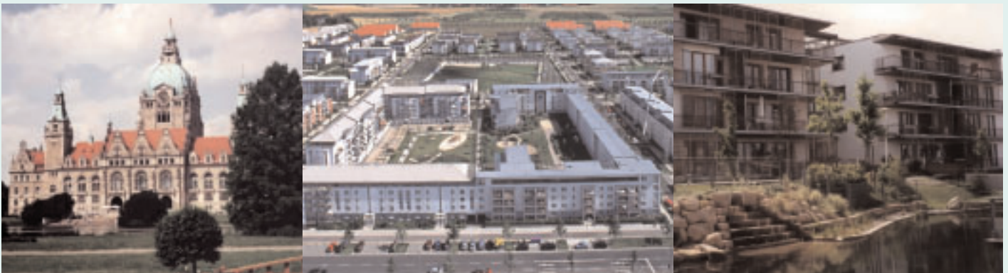
A green paradise within the city: In Hannover, 6,000 eco-friendly flats are under construction.
